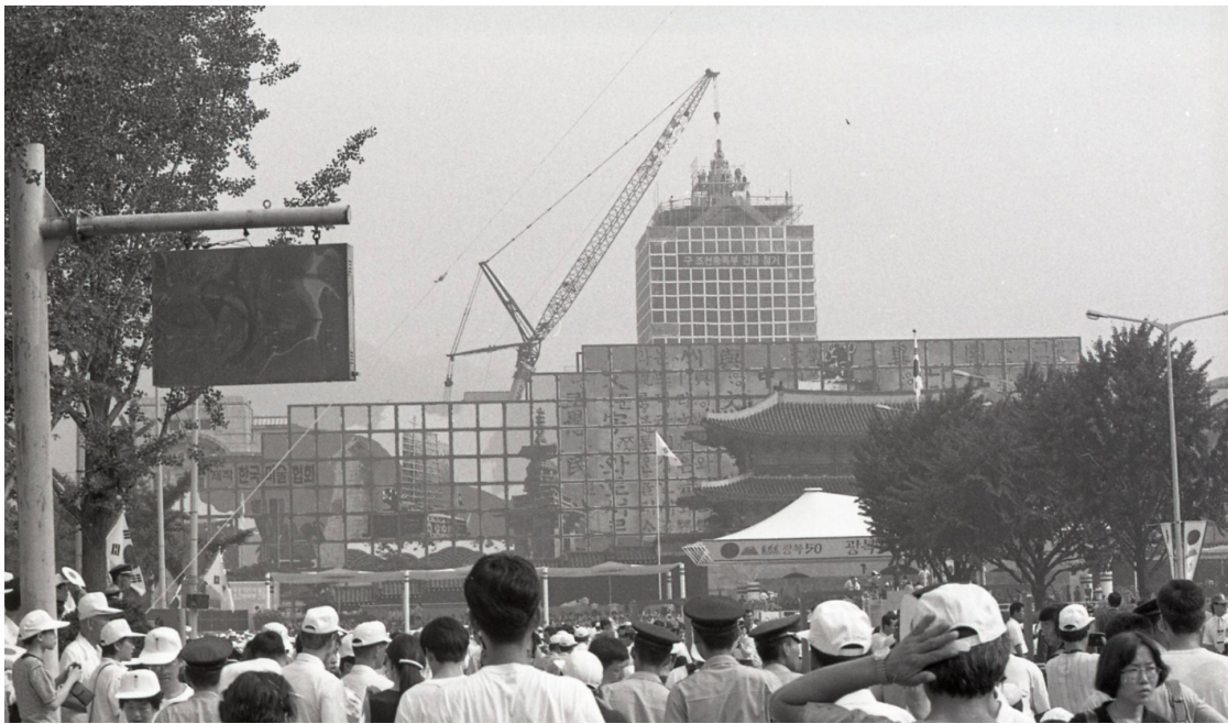
Figure 8.2: Demolition of Joseon-Governor Building (1995)
